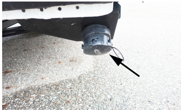
Sewage Drain Outlet (Located beneath the motorhome on the driver side rear.)
