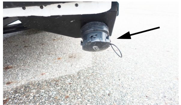
Sewage Drain Outlet (Located beneath motorhome on the drivers side) - Typical View
